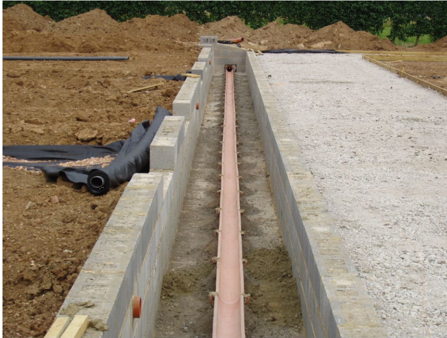
Figure 4: Laying the main drain within the culvert at East Malling Water Centre. On the left are 3 (5 x 10m) beds and on the right the forklift access track
