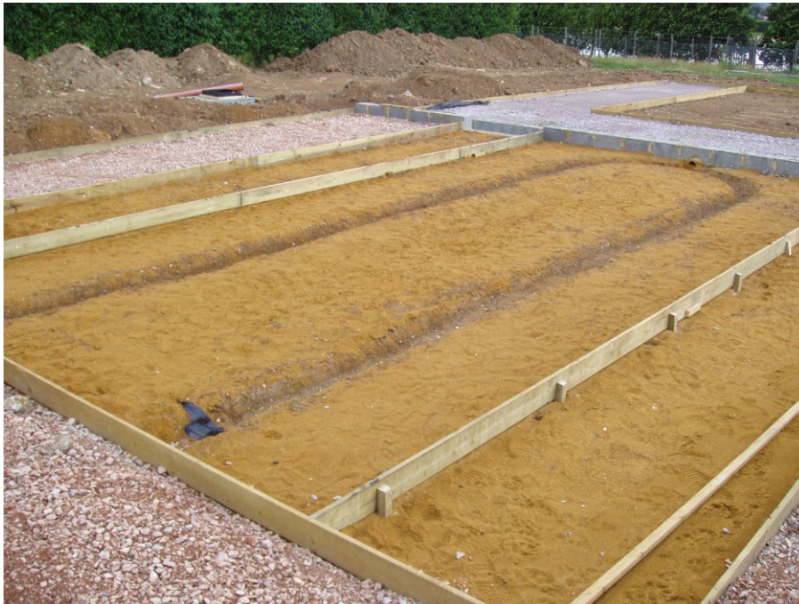
Figure 4: Laying the main drain within the culvert at East Malling Water Centre. On the left are 3 (5 x 10m) beds and on the right the forklift access track
