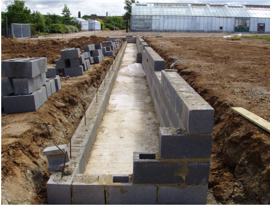
Figure 2: Construction of the main supply and drainage culvert at the East Malling Water Centre
