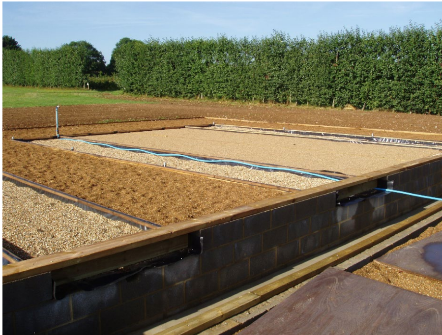
Figure 10: The final stages of bed construction with the installation of water supply at the East Malling Water Centre
