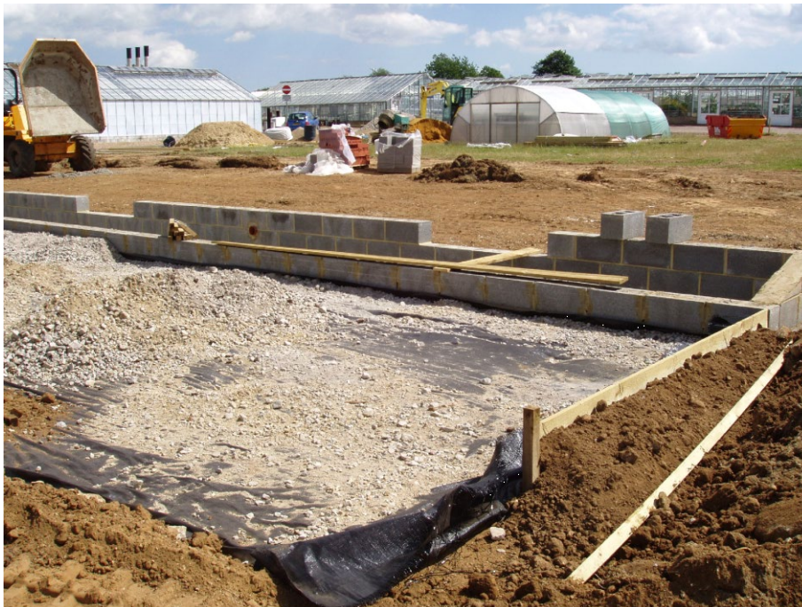
Figure 2: Construction of the main supply and drainage culvert at the East Malling Water Centre
